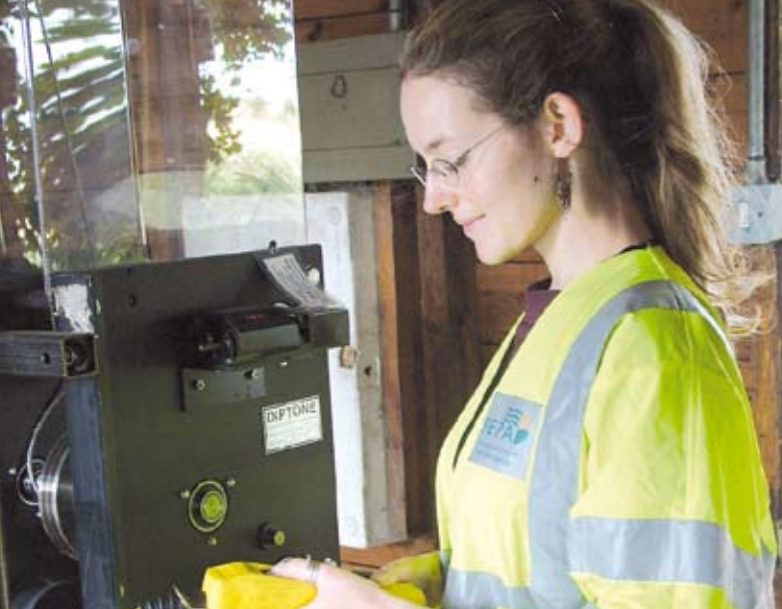
Checking instrumentation inside a gauging station of the Scottish Environment Protection Agency (Photo by courtesy of SEPA, 2003)
